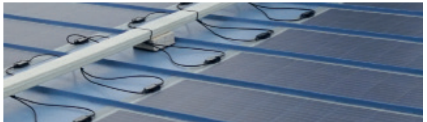
Fig. 10: Example of a cable tray, which is distanced from the roof
